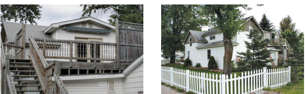
401 WATER STREET • EAST JORDAN
